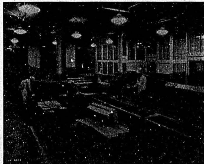
RLM Standard Reflector Domes, used in this food-processing plant, provide a satisfactory level of well distributed lighting.
